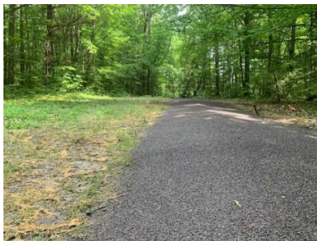
Trail crowned to drain water.
