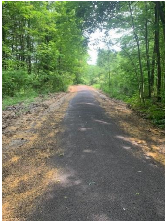
New ditch creation.
